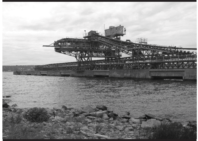
National Gypsum Dock Rehabilitation Dartmouth, Nova Scotia
