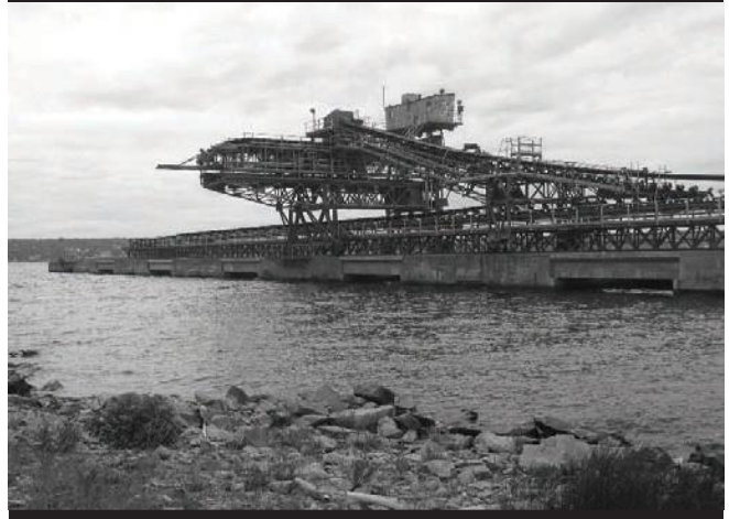
National Gypsum Dock Rehabilitation Dartmouth, Nova Scotia
